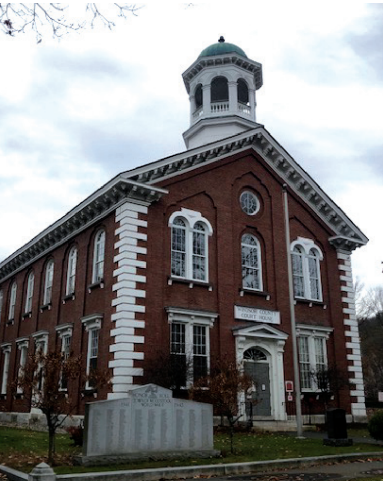
Windsor County Court House, Vermont
